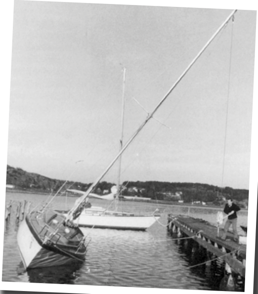
Heeling test in 1965. The righting moment of the boat is measured at 30° heel.
